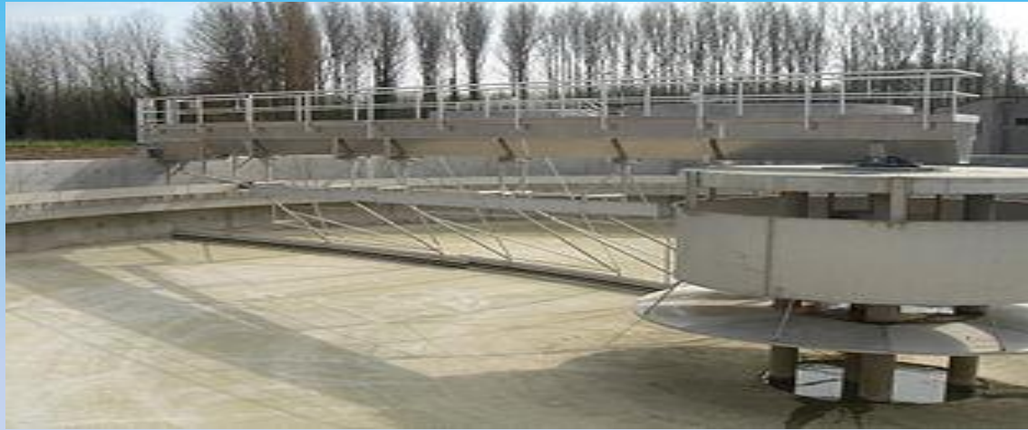
An empty sedimentation tank at the treatment plant
